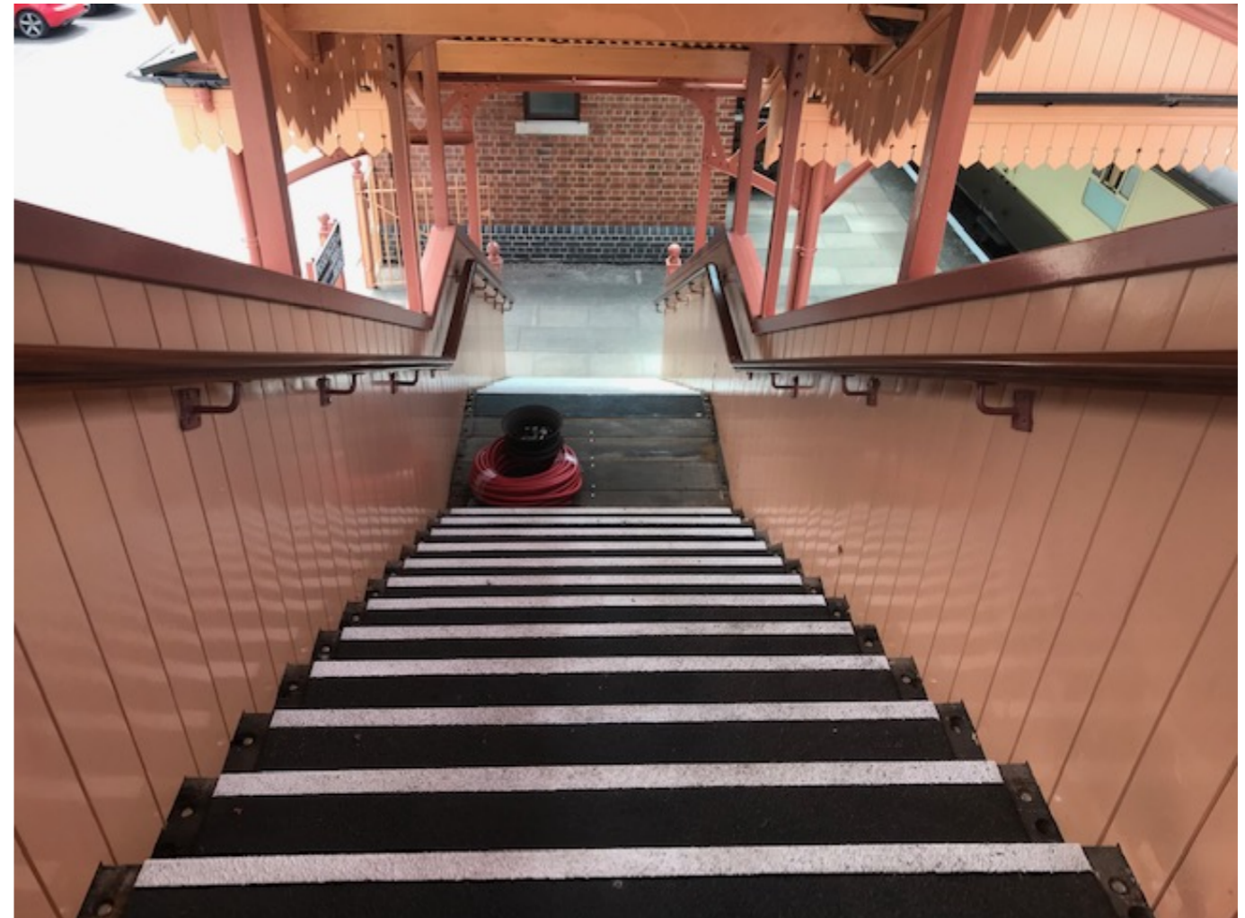
Reference: UI-44714-555 Broadway Footbridge - Access
