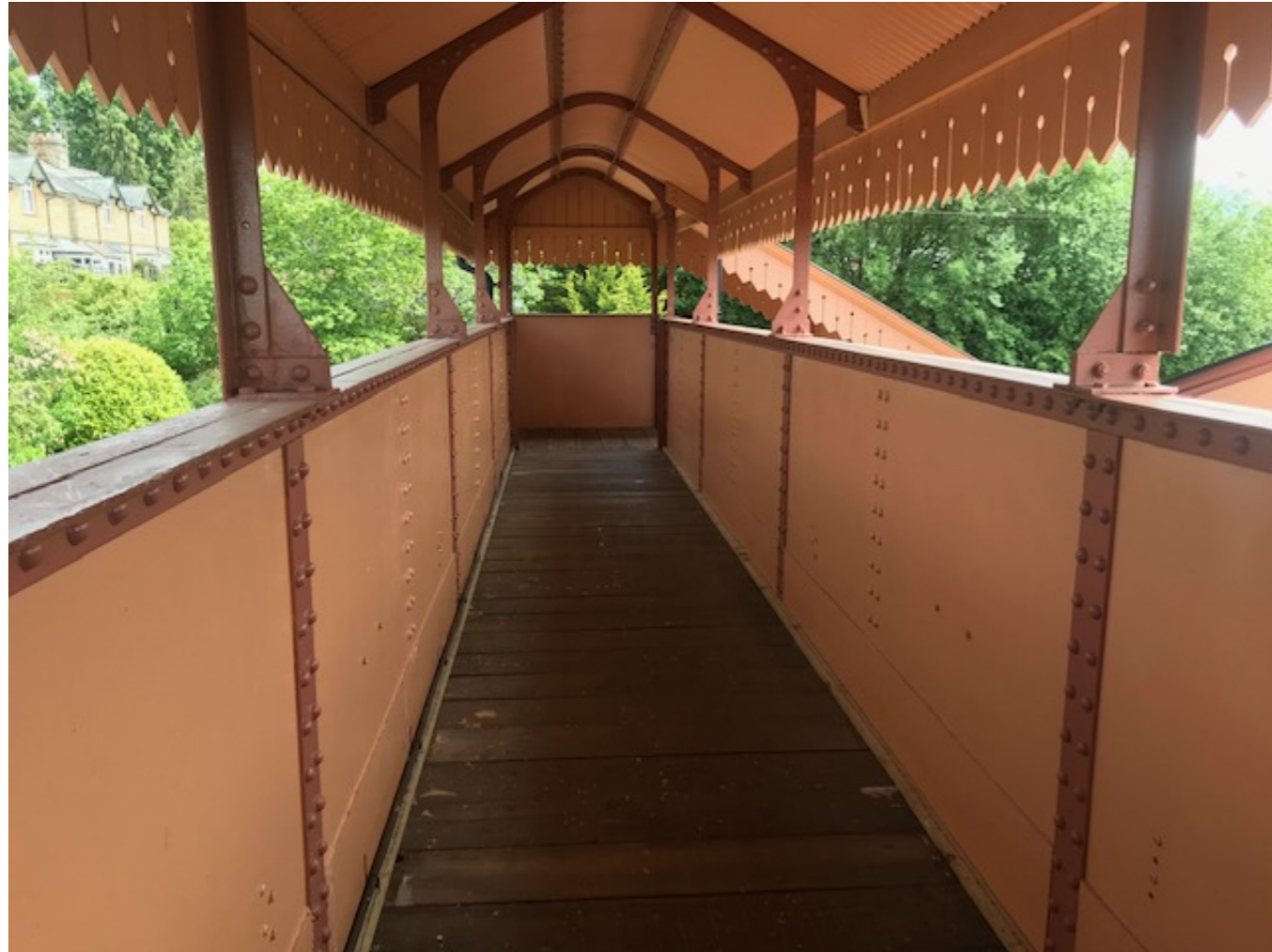
Reference: UI-44714-370 Broadway Footbridge - Main Section
