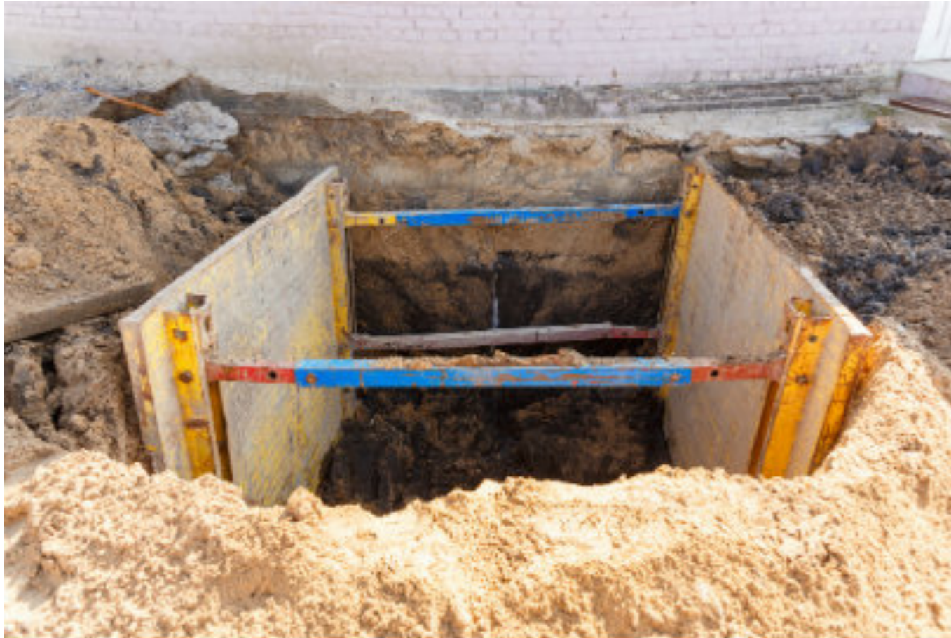
Reference: UI-44519-481 Trench shuttering example -
