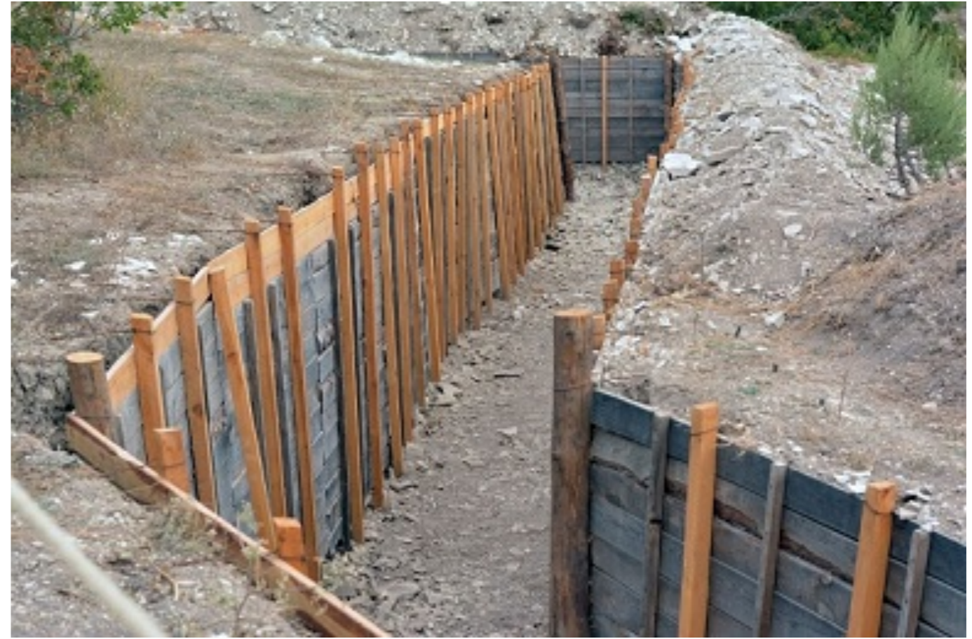
Reference: UI-44519-552 Trench shuttering example -
