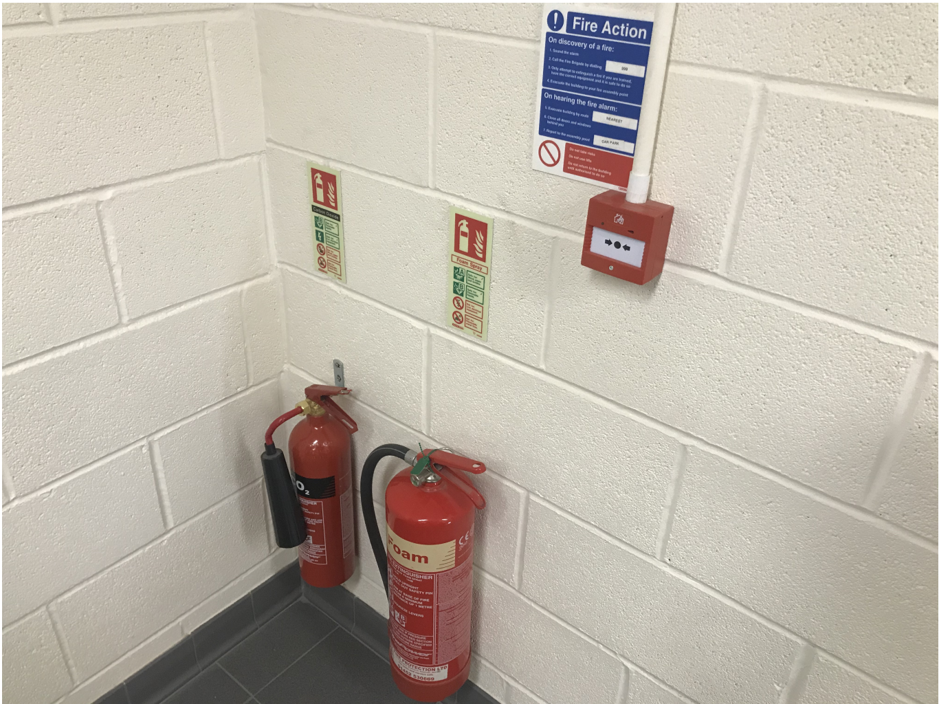
Reference: UI-44313-975 Fire Extinguishers and Alarm Points -
