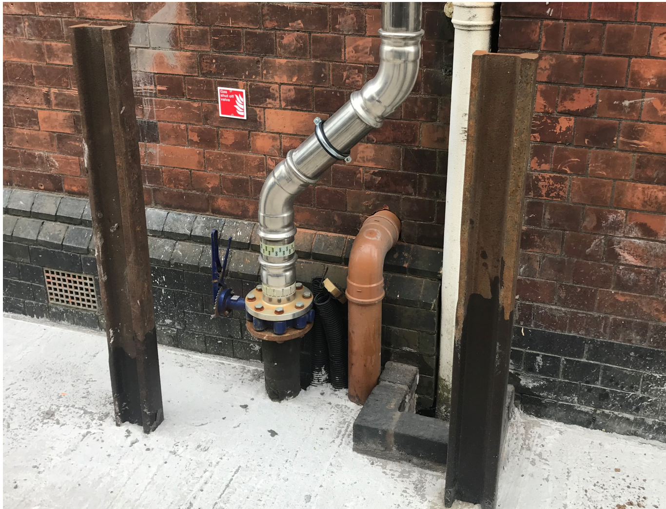
Reference: UI-44313-217 Gas Main and Isolation Valve -
