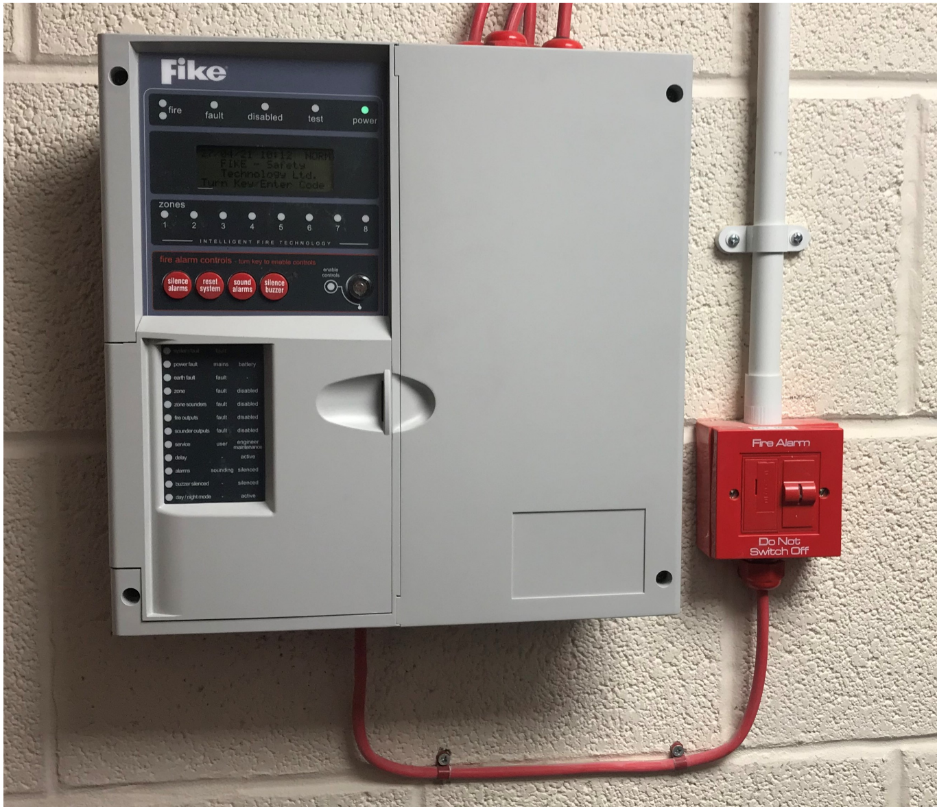
Reference: UI-44313-991 Fire System Panel -
