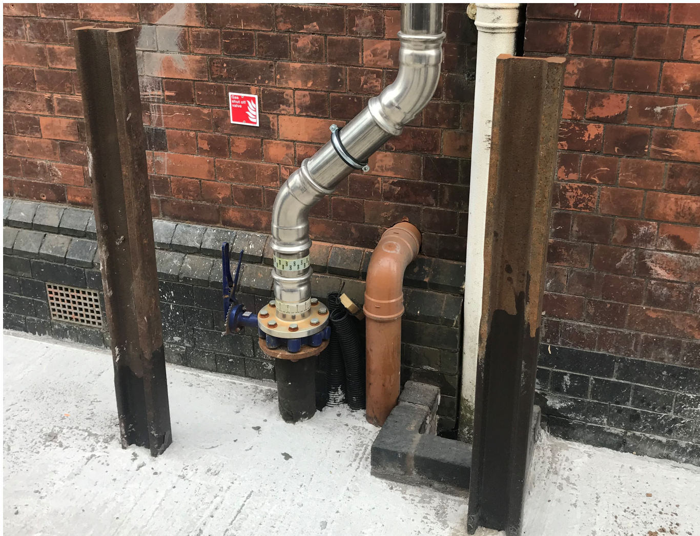
Reference: UI-44313-217 Gas Main and Isolation Valve -
