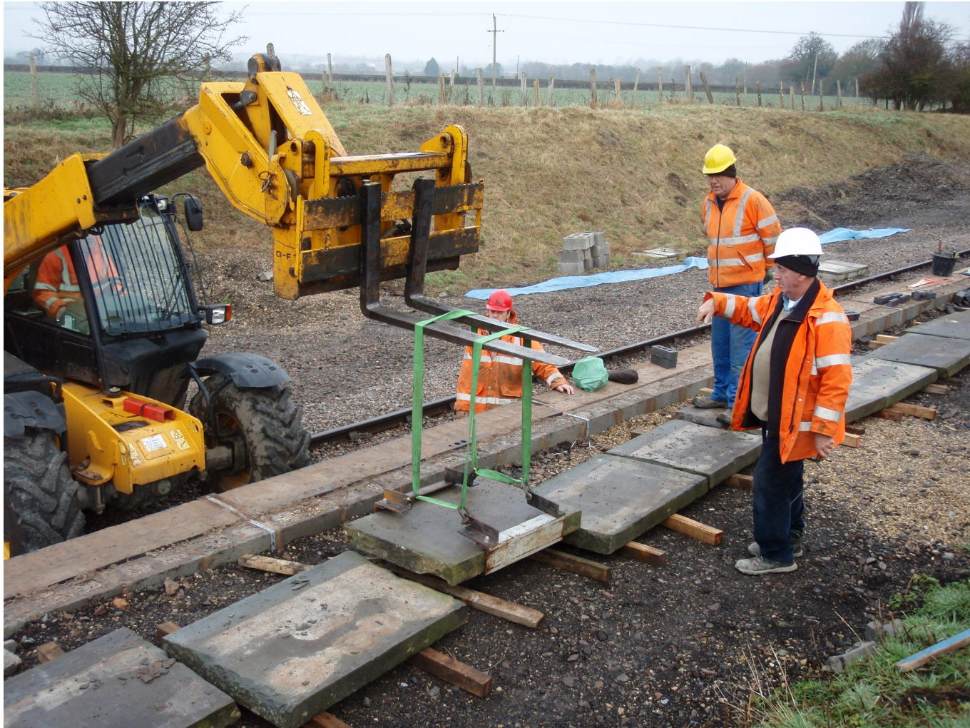
Reference: UI-44434-225 Positioning slabs with a FLT -
