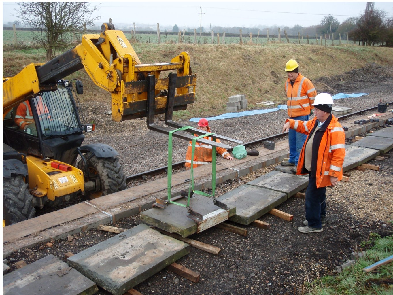
Reference: UI-44434-225 Positioning slabs with a FLT -
