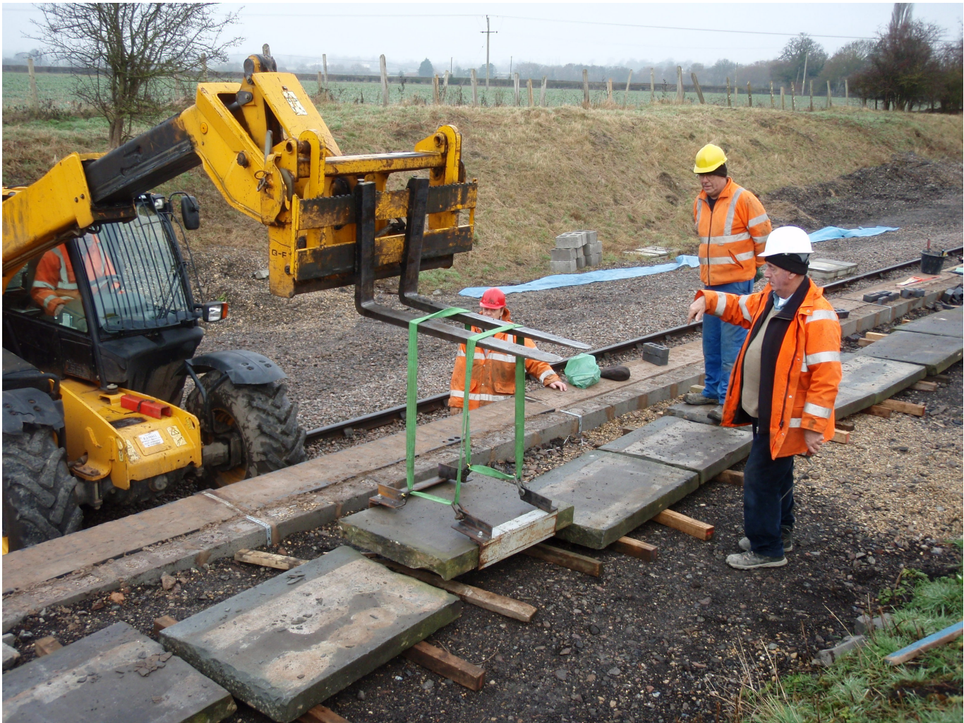
Reference: UI-44434-225 Positioning slabs with a FLT -
